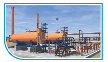
uninterrupted operation in the Far North. Application of 5 MW PPTB unit is economically profitable not only because of the high specific capacity (reduction in the number of used vehicles), but also because of the unique thermodynamic compactness -building area per one unit in comparison with existing analogs is reduced from 272 m<sup>2</sup> to 84 m<sup>2</sup>, which significantly affects the value of the CMP.
